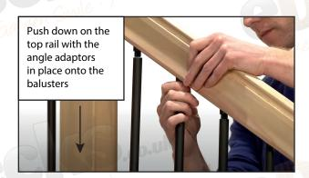
7. Then starting at one end line up the balusters with the angle adaptors in the top pre-drilled rail, moving across the length and pushing the top rail down.
