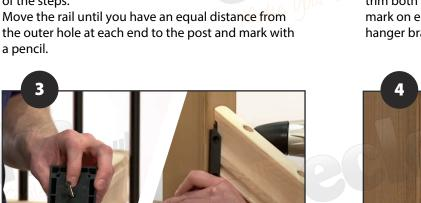
3. Attach the rail hanger brackets to the end of the pre-drilled rails.
