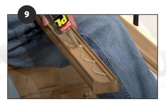
9. If adding the optional cap rail place over the edge of the stairs and mark the same as the pre-drilled rails in step 1, cut the cap rail along the marked line, apply the high-quality pink grip adhesive (sold separately) into the groove of the cap rail.
