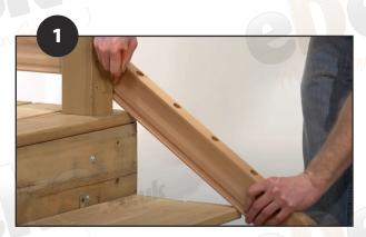
1. With your posts in place simply centre the pre-drilled rail between the two posts, on the edges of the steps.
