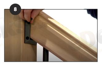
8. Now affix the top rail hanger brackets at each end to the posts, like you did for the bottom rail in step 3.
