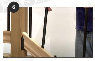
6. The traditional balusters fit over the angle adaptors, place all balusters on the adaptors.
