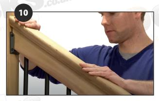
10. Fix the cap rail in place then clamp until the adhesive sets
